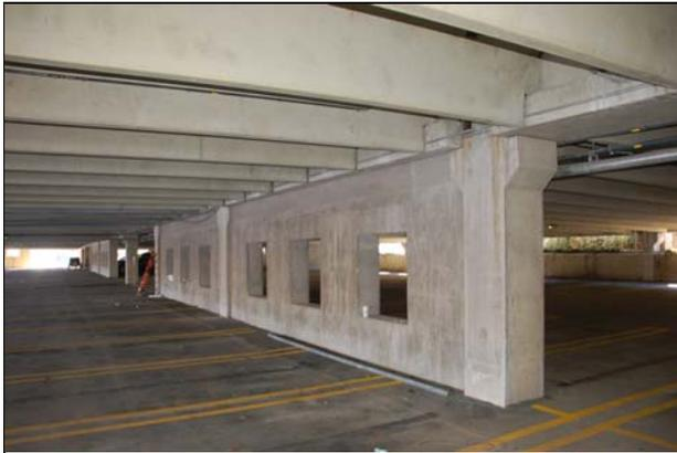
New Cast in Place Concrete Shearwall
