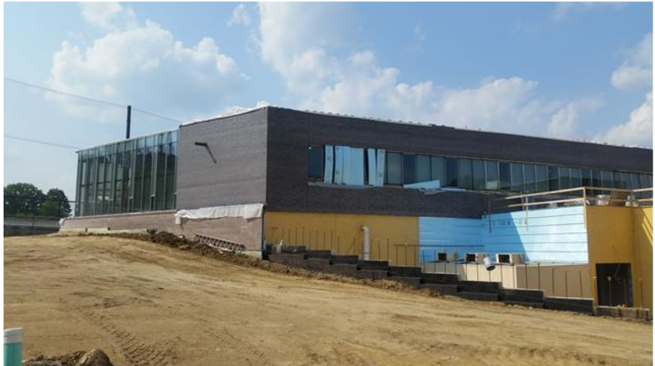
Top drawing shows the site with the first floor half at grade and half below. Bottom Image: Example of the sloping site. (photo © MGA Partners, Architects)
