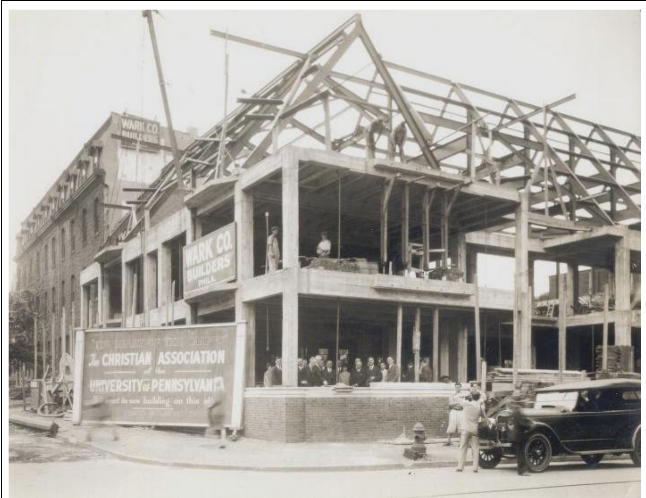
Construction of the ARCH circa 1928 (photo courtesy of the Christian Association)
