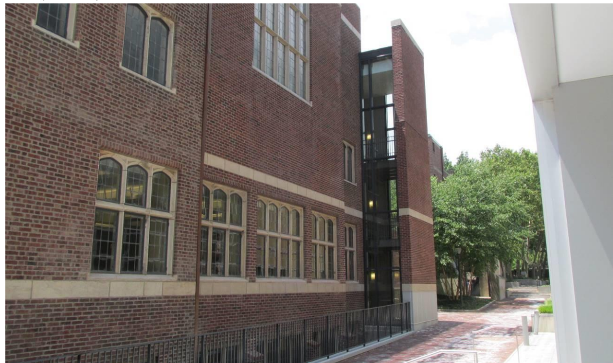
A new stair tower was added to the northern side of the ARCH (photo © Keast & Hood)
