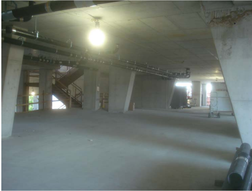
Photograph 3 – SLOPED COLUMNS BETWEEN PARKING LEVEL 4A AND LEVEL 6
