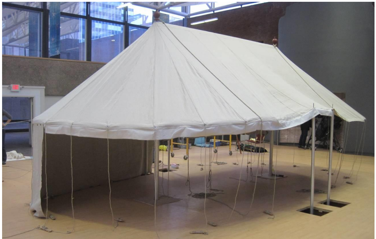
Keast & Hood designer Alex Stadel adjusts the support structure. (photos © Keast & Hood)
