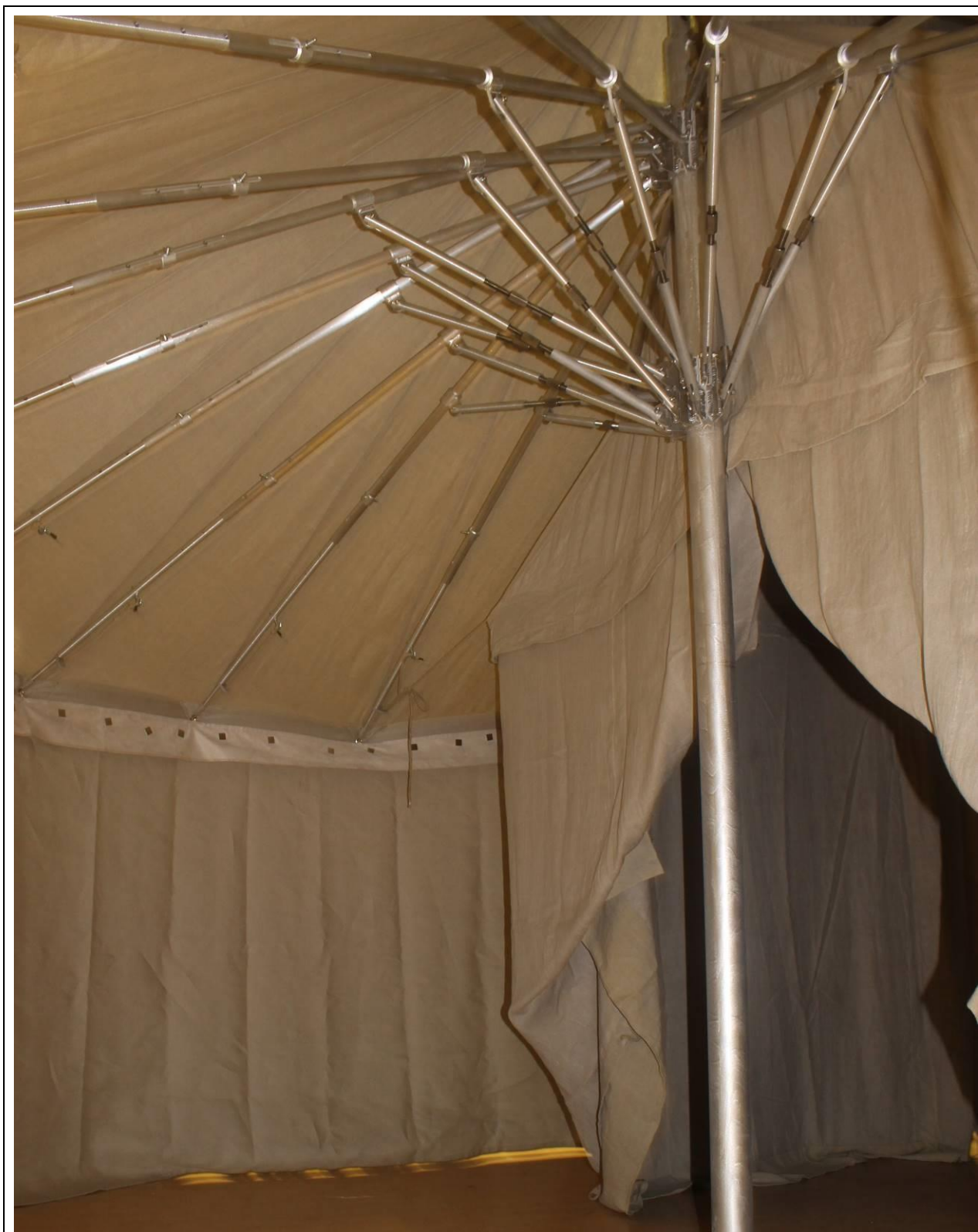
A view from the inside of the tent exhibits the structure's ribs and subtent. (photo © Keast & Hood)
