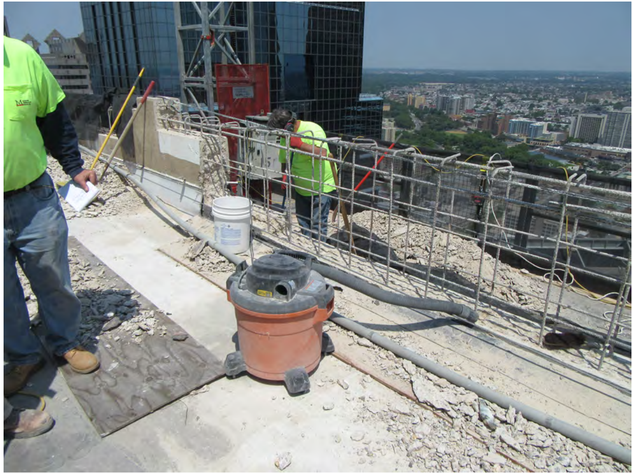
Parapet repairs at roof level along Market Street
