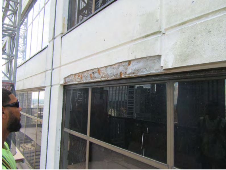
BEFORE: Concrete repairs in process
