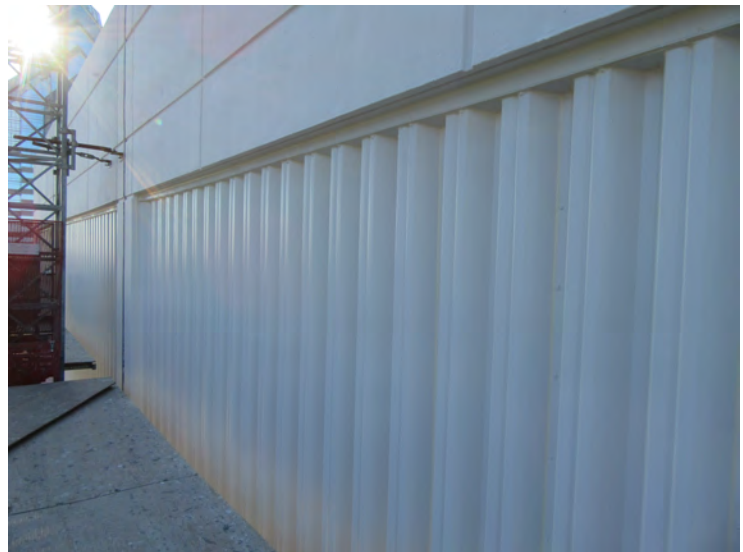
AFTER: Condition of building after repairs and coating
