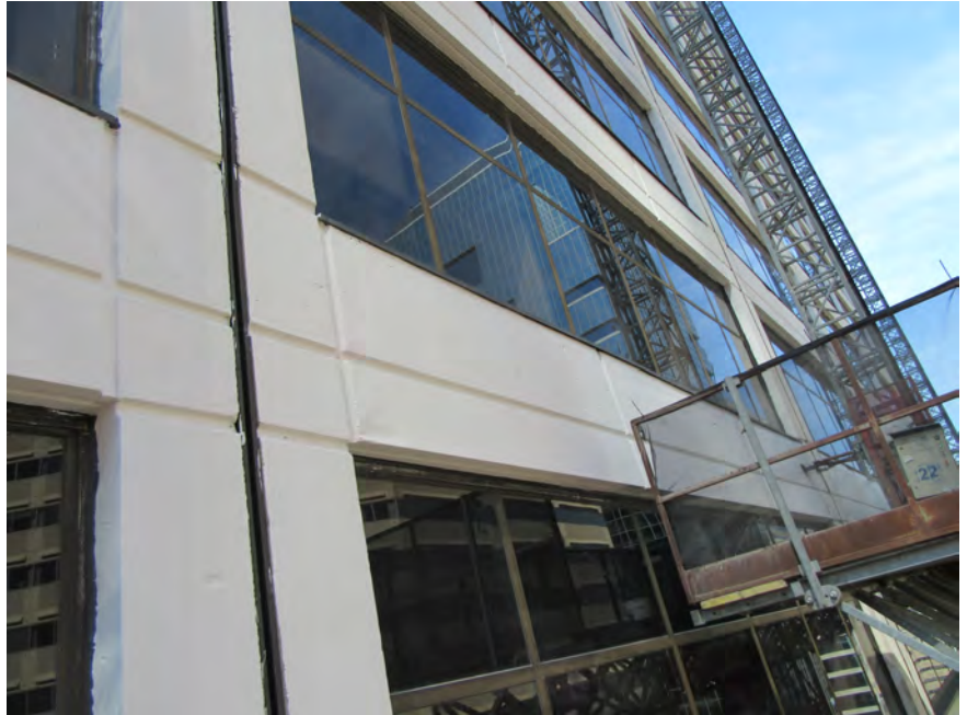
AFTER: Completed concrete repairs with coating
