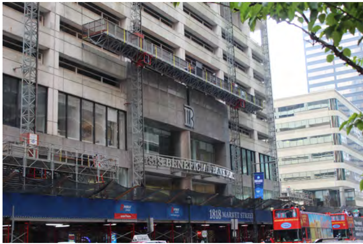
Mast Climbers - North Elevation
