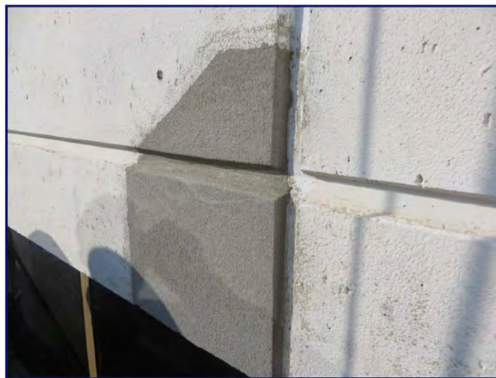
Completed concrete repair before coating
