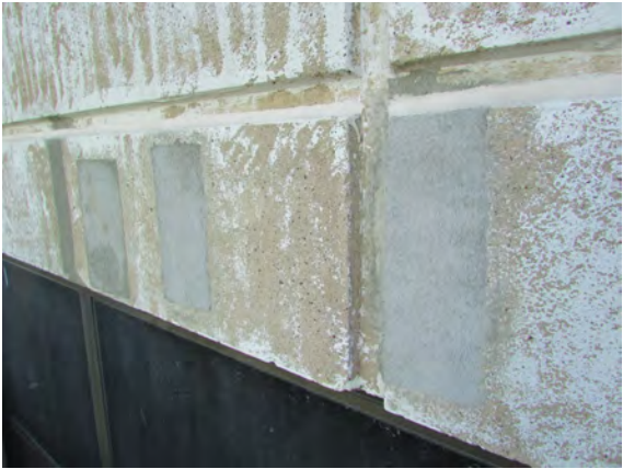
Completed concrete repairs before coating
