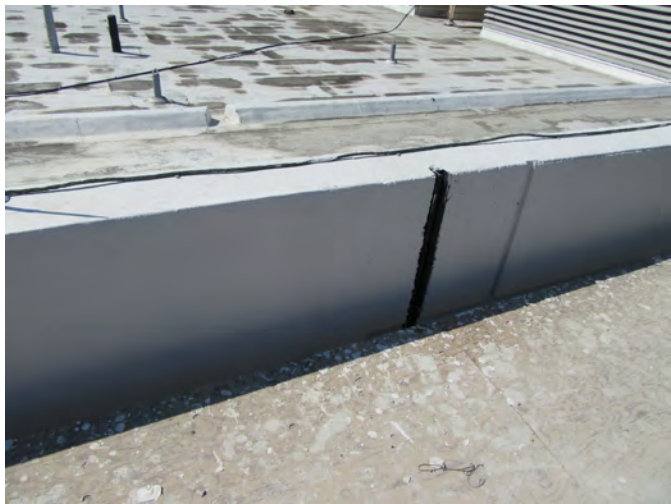
Completed concrete repairs with coating
