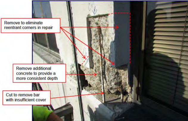
Column corner repair with instruction
