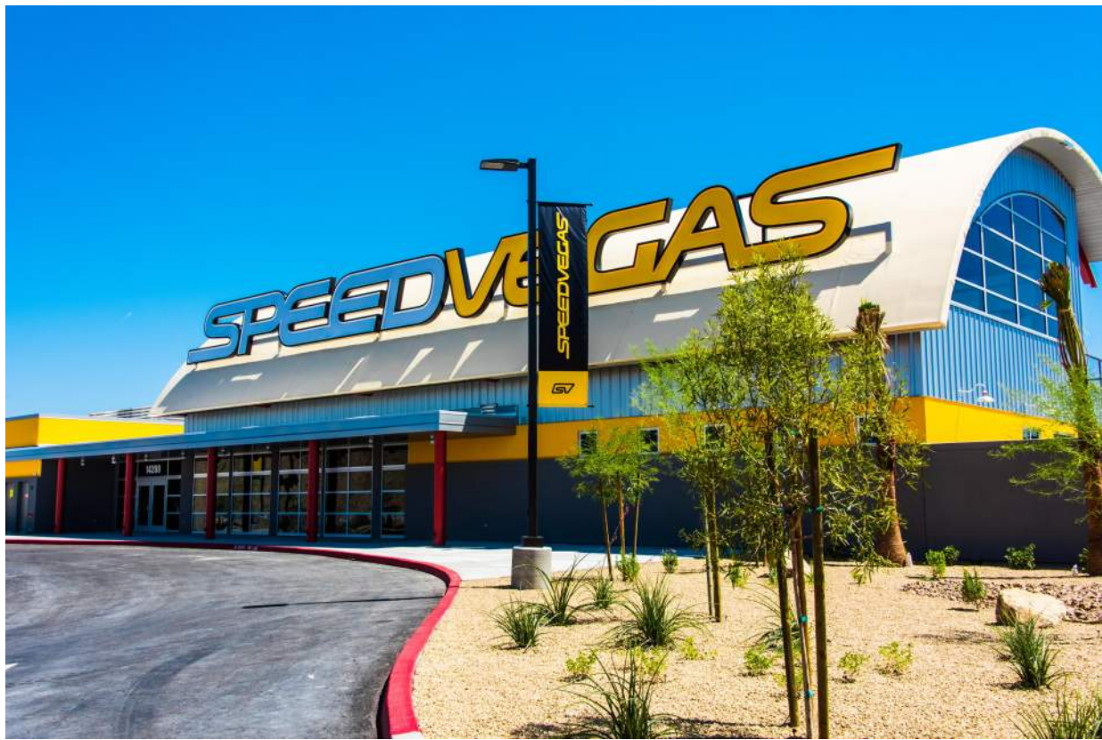
Exhibit A (Above): Exterior view of the completed race course clubhouse showing the rear of the fabric roof, Speed Vegas sign, and the leading edge of the curved eave (right background).
