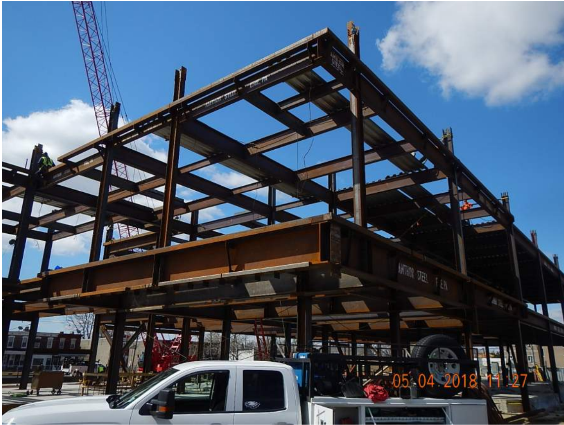
2 ND and 3 RD floor steel.
