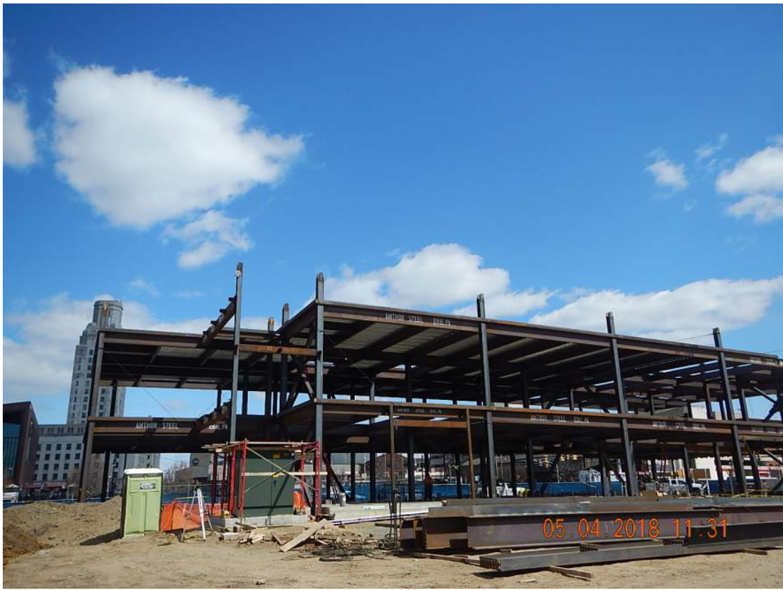
Steel being erected.
