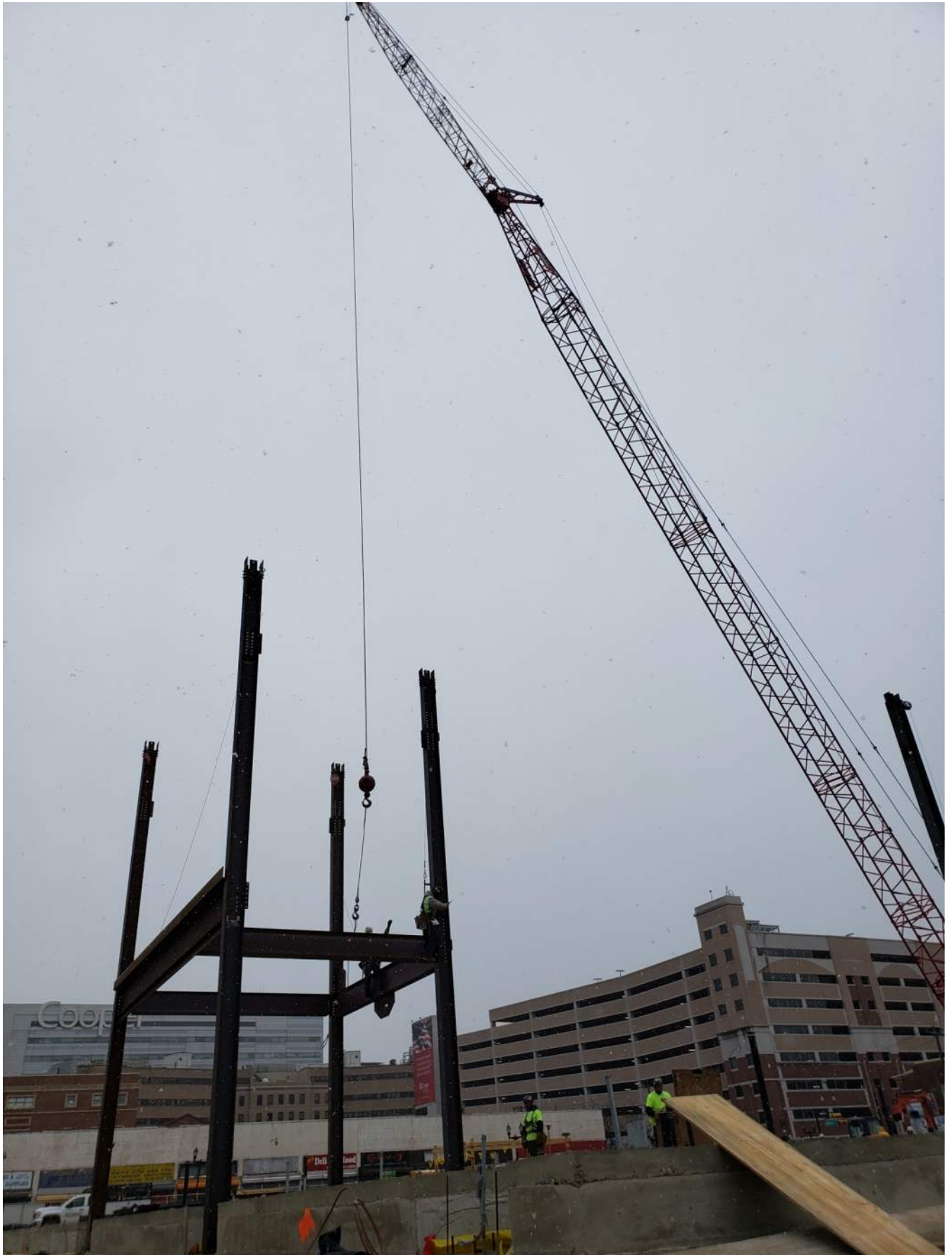
First steel being erected.
