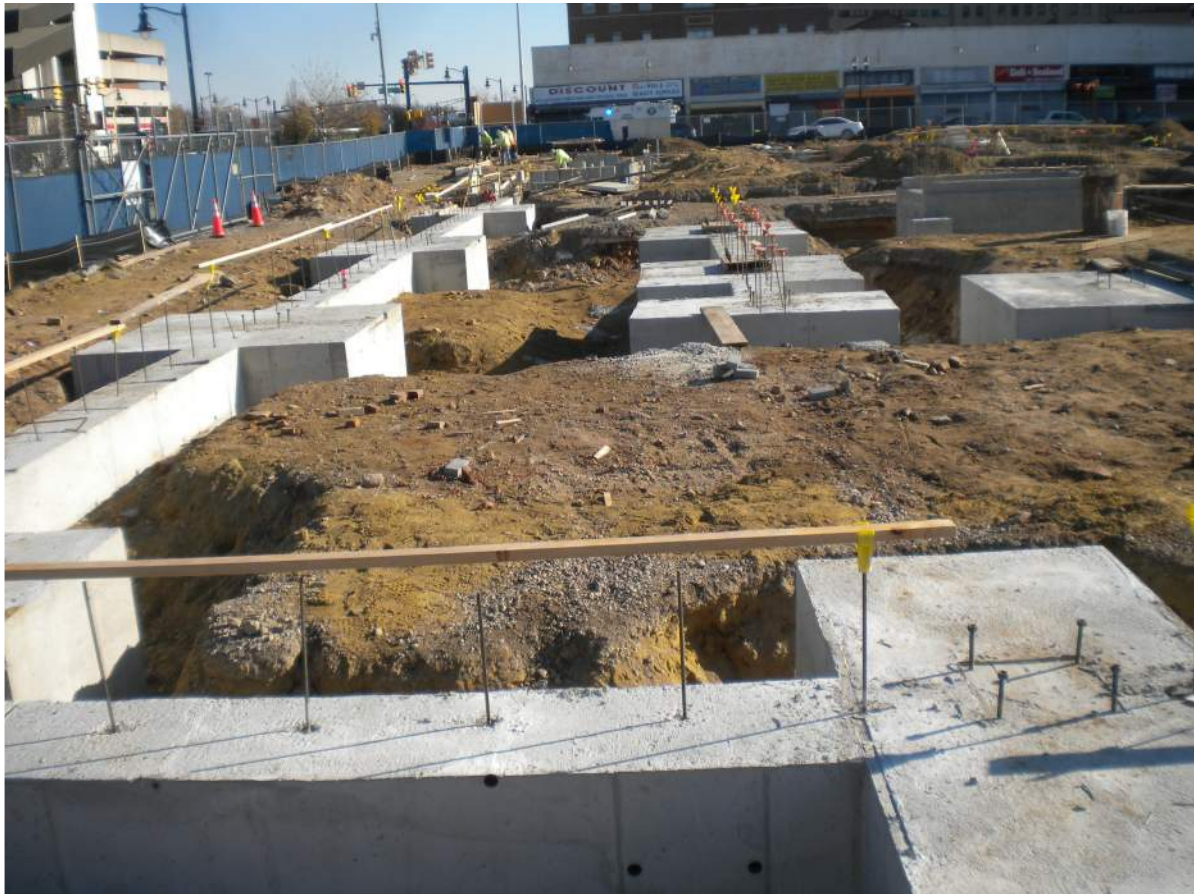
Pile caps and grade beams.
