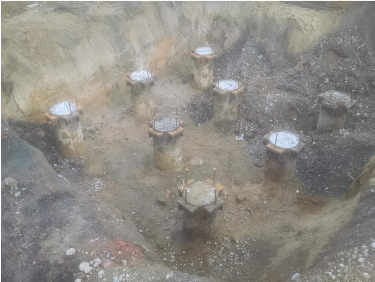
Installed piles with uplift anchors.
