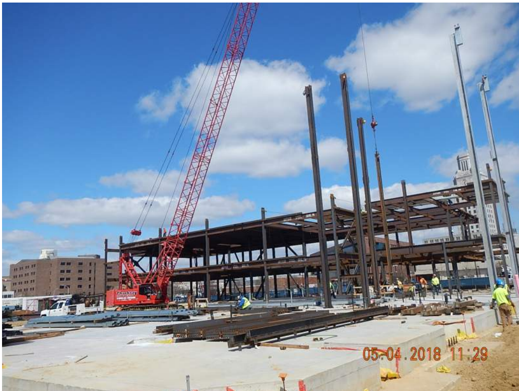
Crane, north leg steel, and south leg slab on grade.
