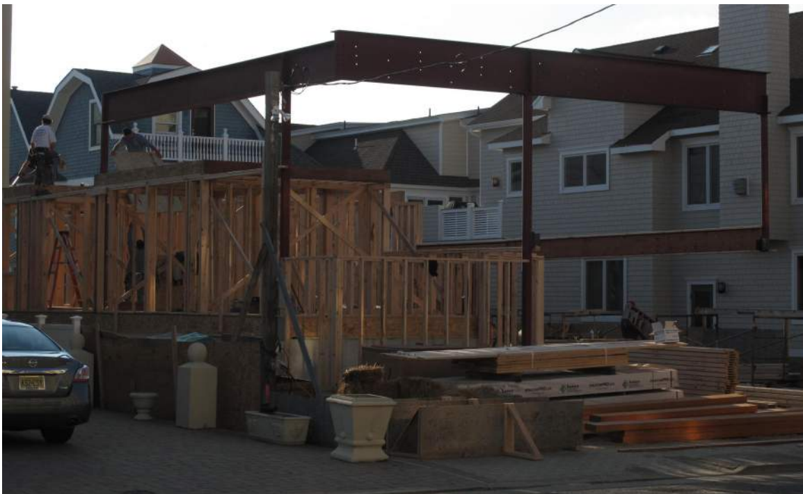
Exhibit C (Above): Construction photo showing wood-frame cantilever over future garage space assisted by steel transfer girder and hanger support for 2nd floor. Exhibit D (Below): Construction photo with steel transfer frame highlighted with HSS hanger support for cantilevered floor.
