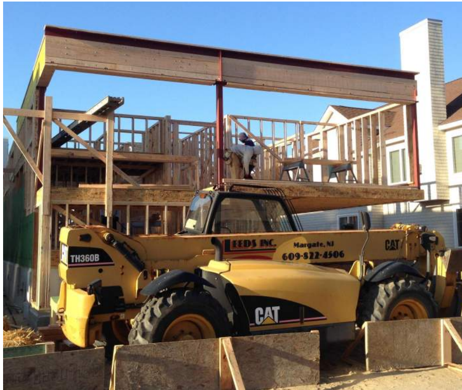
Exhibit C (Above): Construction photo showing wood-frame cantilever over future garage space assisted by steel transfer girder and hanger support for 2nd floor. Exhibit D (Below): Construction photo with steel transfer frame highlighted with HSS hanger support for cantilevered floor.
