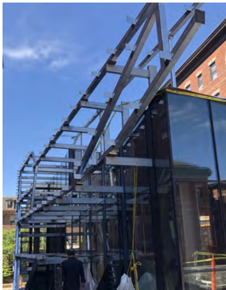
Veil Framing with Curtain Wall
