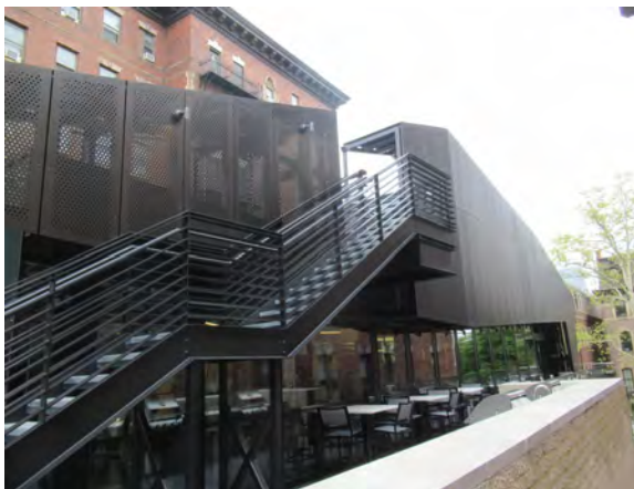
BELOW: Exterior Stairs from 2nd Floor Terrace to 3rd Floor Terrace
