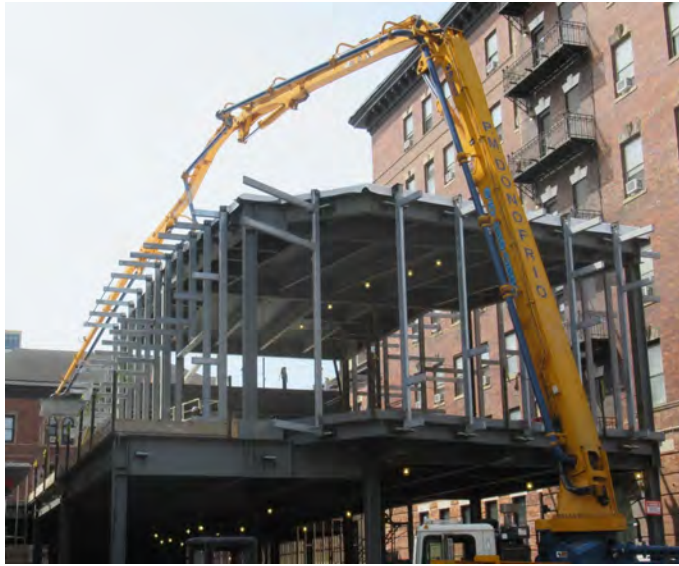
ABOVE: Installation of the Veil Framing
