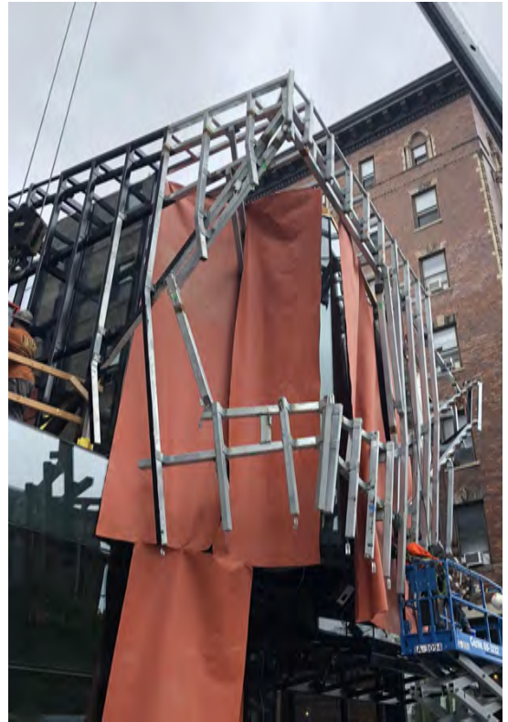
RIGHT: Installation of Veil Framing with Corner Opening & Purlin Sub-frame System
