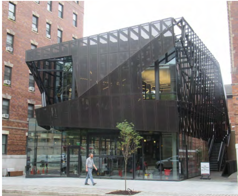
North Facade along Chestnut Street - Veil Panels Partially Installed
