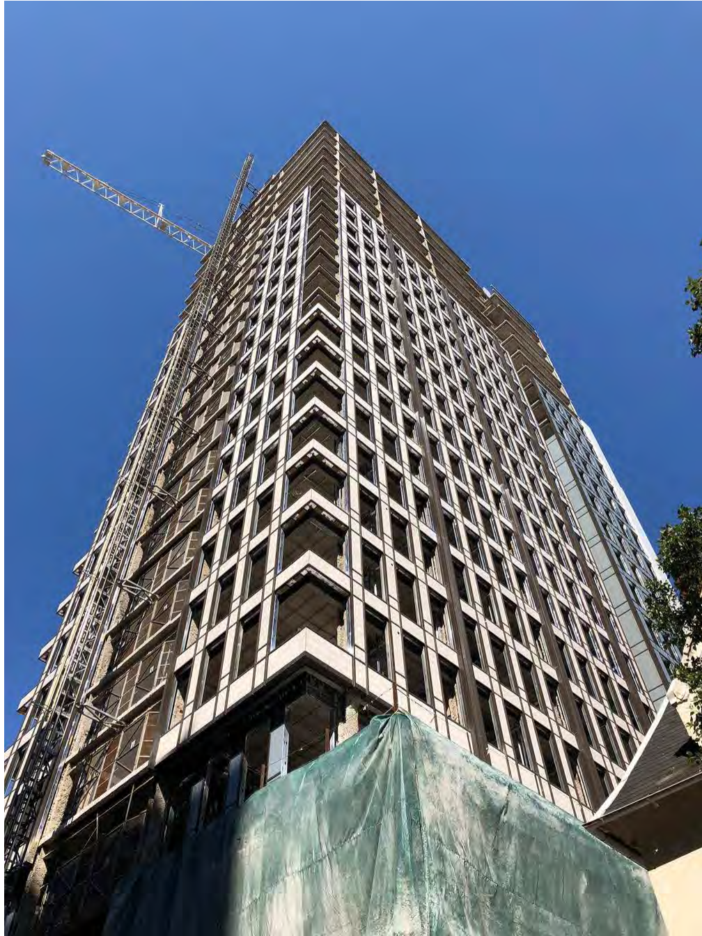
The Harper topped off as only the second building in Philadelphia to use grade 65 steel.
