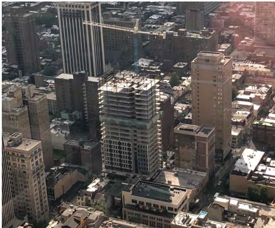
View of the Harper under construction from One Liberty tower.
