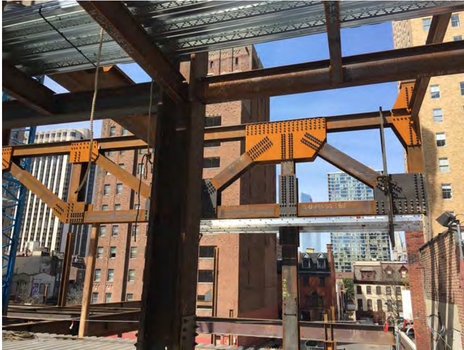
One of (5) transfer trusses over the retail level, grade 65 steel members.
