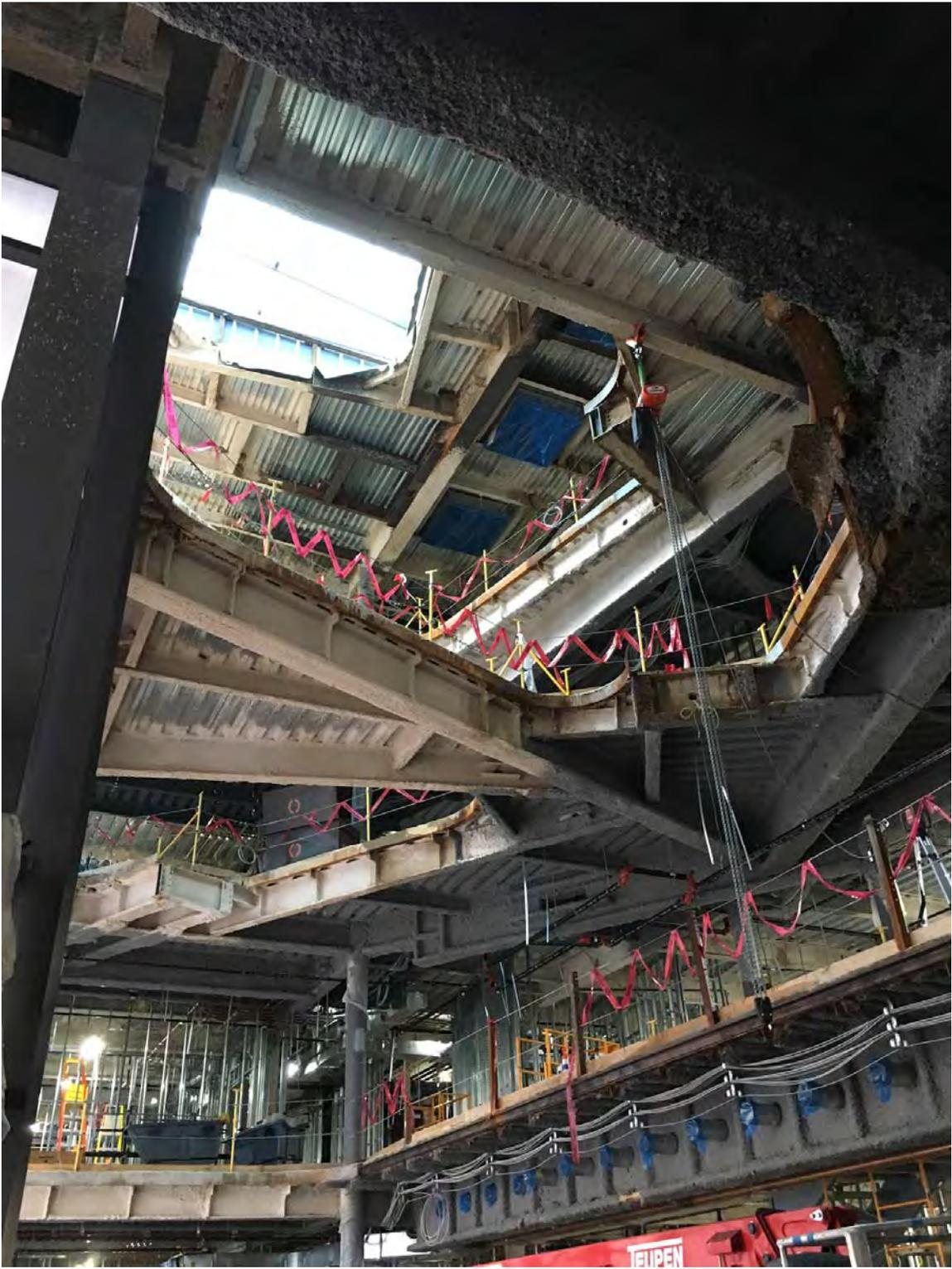
Complex atrium framing forming organically shaped floor openings, sized for vibration control of the atrium stairs, and showing beam web openings.
