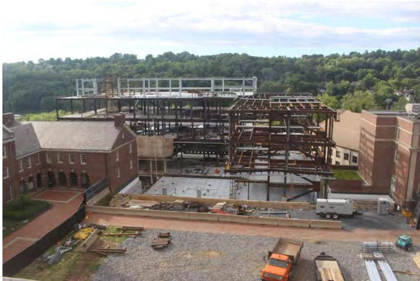
Steel superstructure erected with formwork for 16" cast-in-place concrete slab to support courtyard extension on to building
