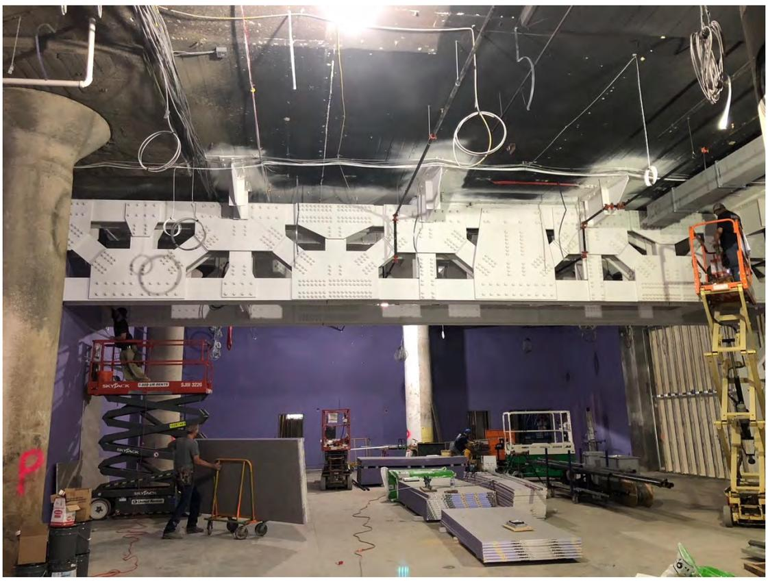
Steel truss supporting the transfer girder which supports 10 floors above.
