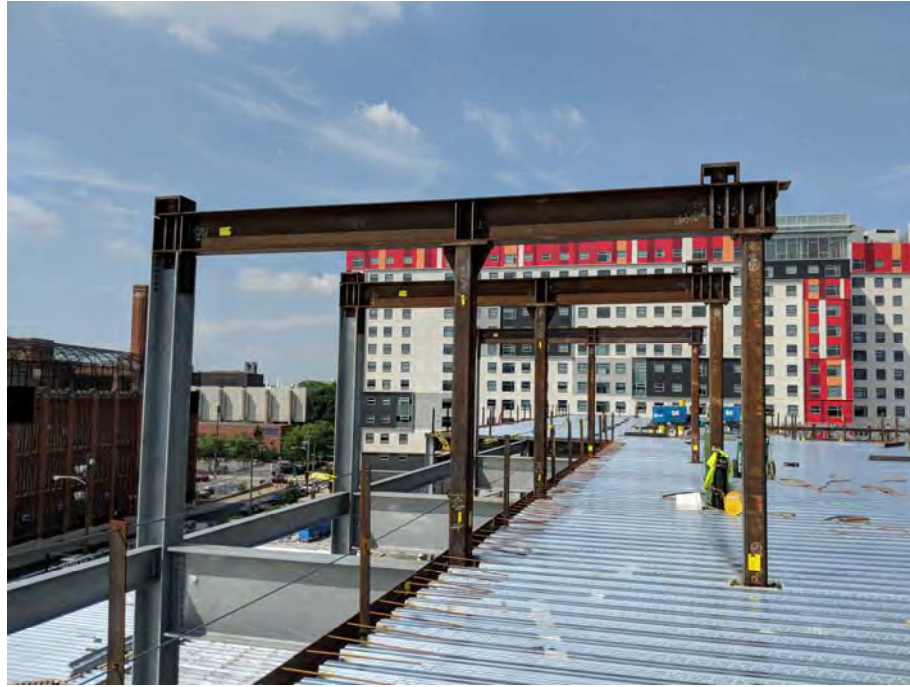
6 th Floor Level Transfer Framing above 5 th Floor Primary Transfer Level with exposed columns against curtainwall façade
