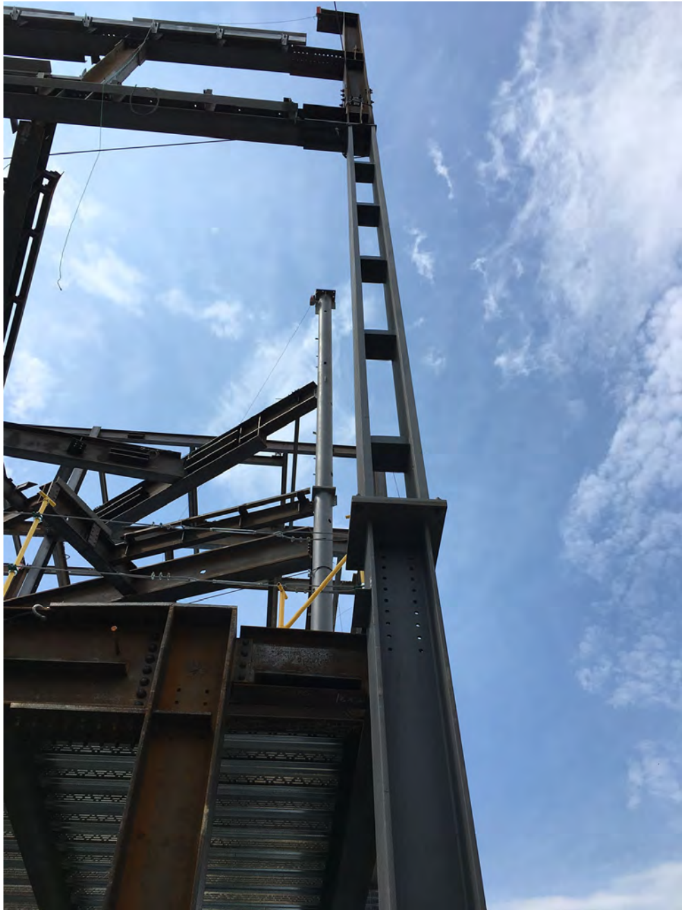
Custom designed ladder column with stitch plates, supporting the Vierendeel truss.
