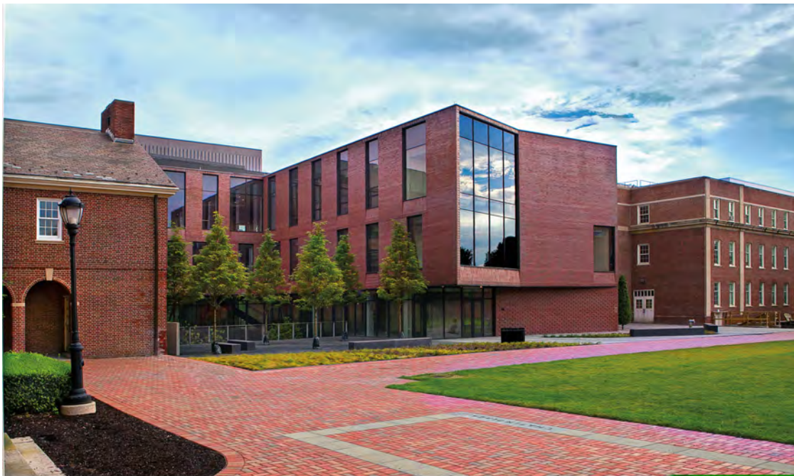
Current view of the RISC from Anderson Courtyard.
