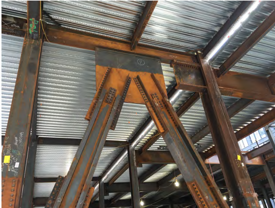
Phase 1 Braced frame with lateral drag connection shown on the upper right to transfer lateral forces from the tower to the podium.
