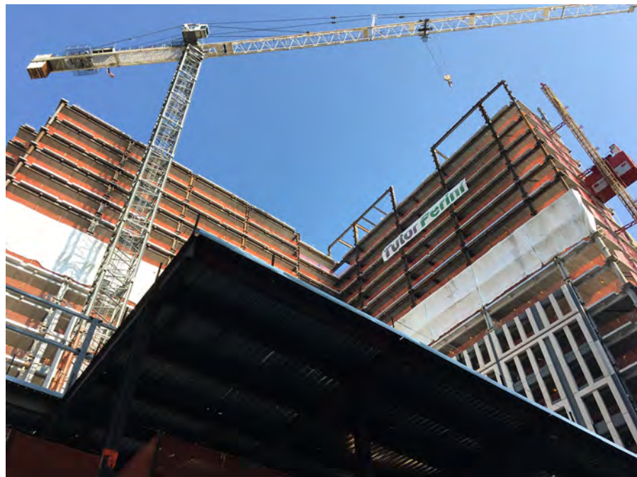
Phase 1 Topping Off
