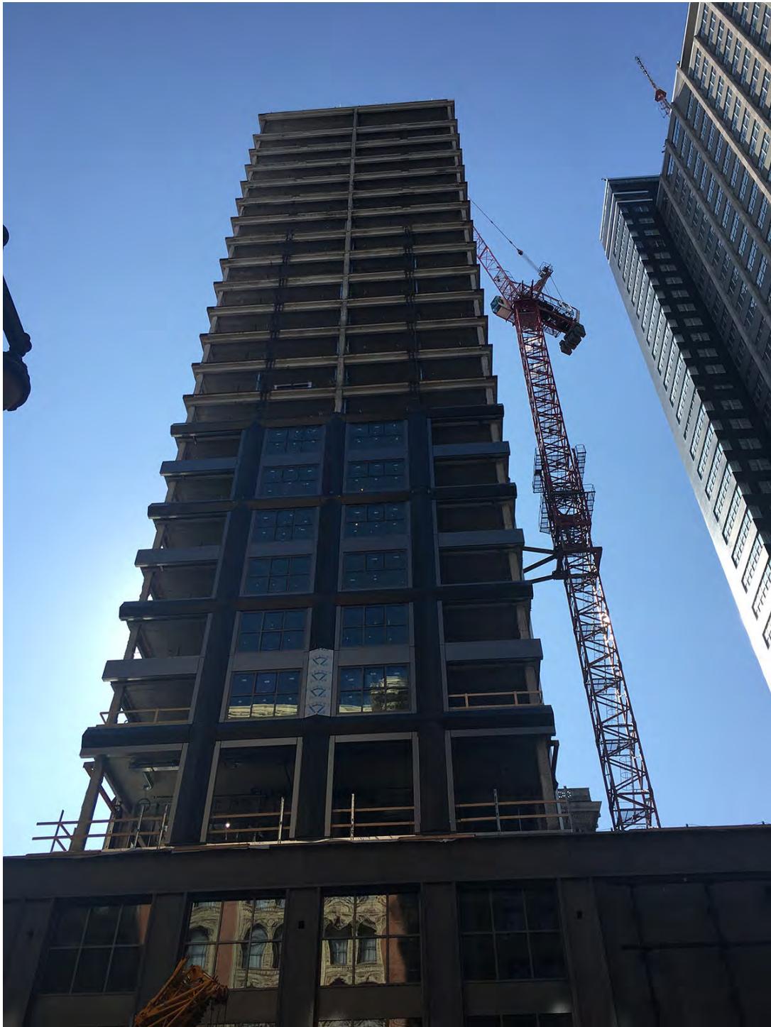
Phase 2 tower Topping Off
