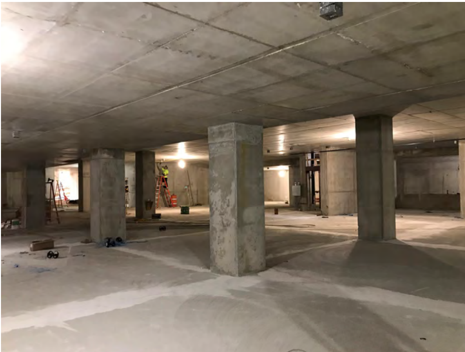
Below ground parking level looking southwest
