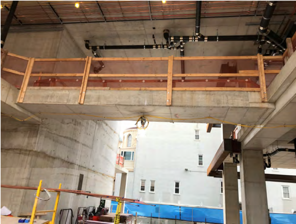
Level 2 bridge looking west
