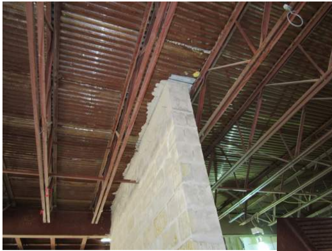
VIEW OF SHEARWALL CONNECTION TO EXISTING SLAB
