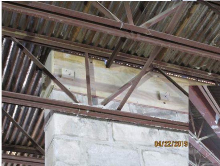
VIEW OF SHEARWALL CONNECTION TO EXISTING SLAB
