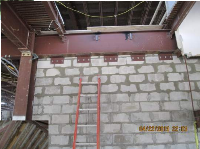
VIEW OF SHEARWALL CONNECTION TO EXISTING SLAB
