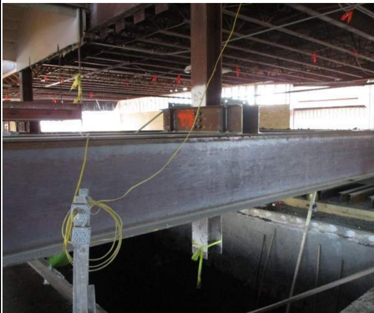
VIEW OF UNDERPINNING PROCESS AT INTERIOR COLUMNS
