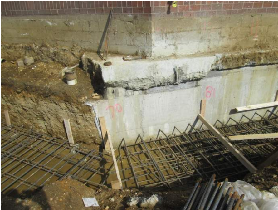
VIEW OF EXTERIOR UNDERPINNING PROCESS AT LOADING DOCK
