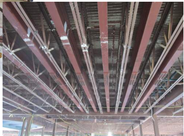
VIEW OF NEW FRAMING BETWEEN EXISTING JOISTS
