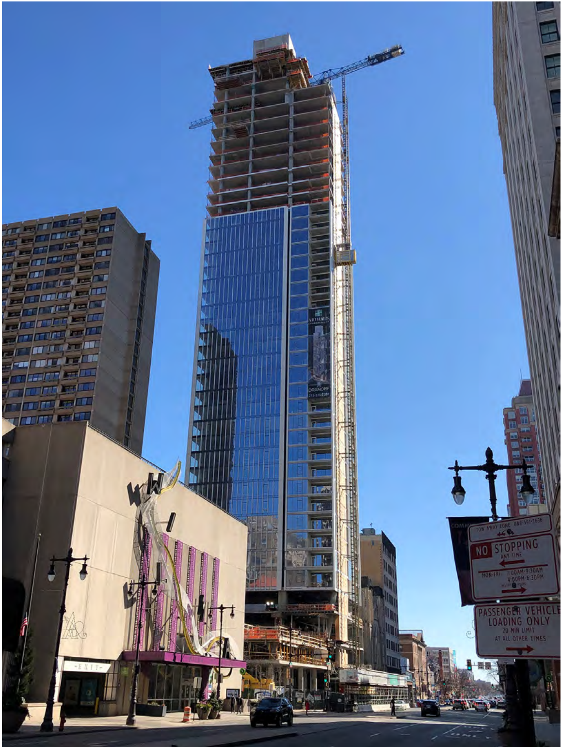
Under construction, March, 2021
