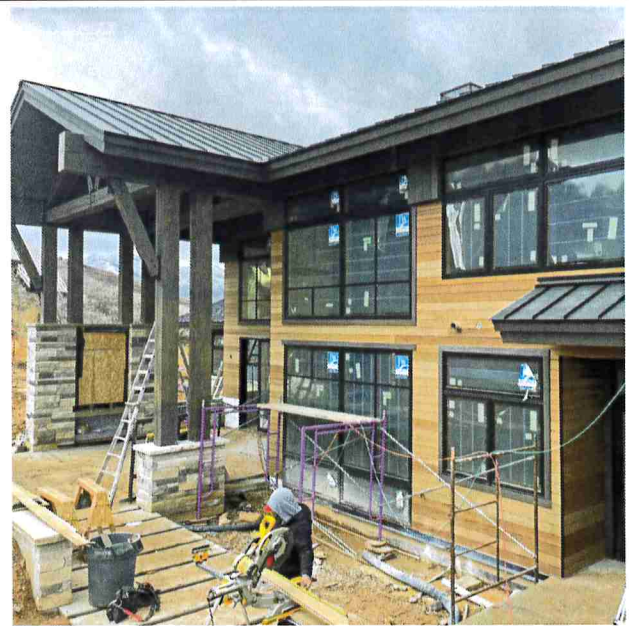
NORTH FACADE OF THE BUILDING WITH CONCRETE PEDESTALS SUPPORTING ROOF OVER COVERED PATIO AREA
