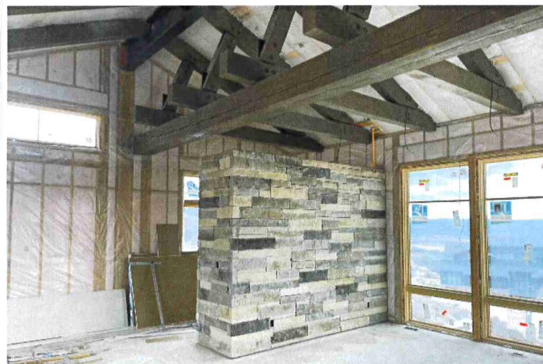
THE VAULTED ROOF FRAMING AT THE KITCHEN AND DINING AREAS.
