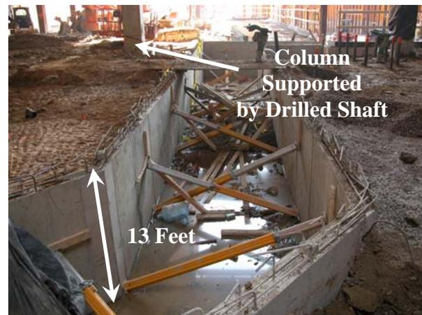
Figure 3 – Below-Slab Utility Trench
