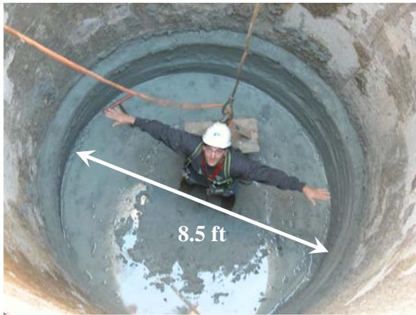
Figure 5 – Drilled Shaft Installation and Inspection
