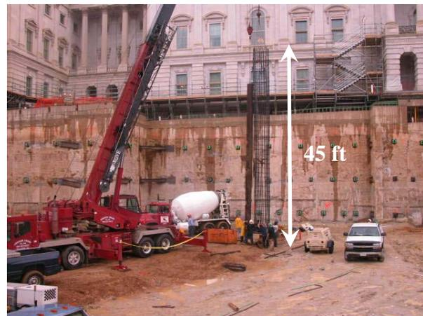
Figure 4 – Drilled Shaft Installation
