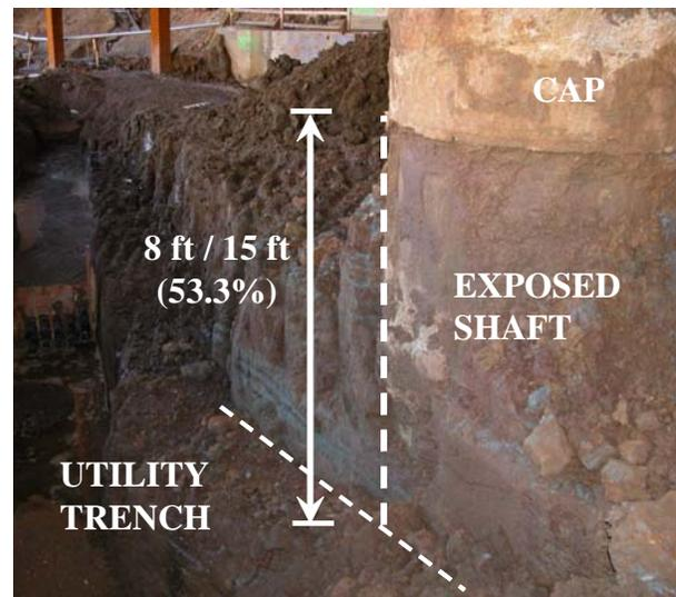
Figure 10 – Exposed Drilled Shaft in Northwest Corner of Site
