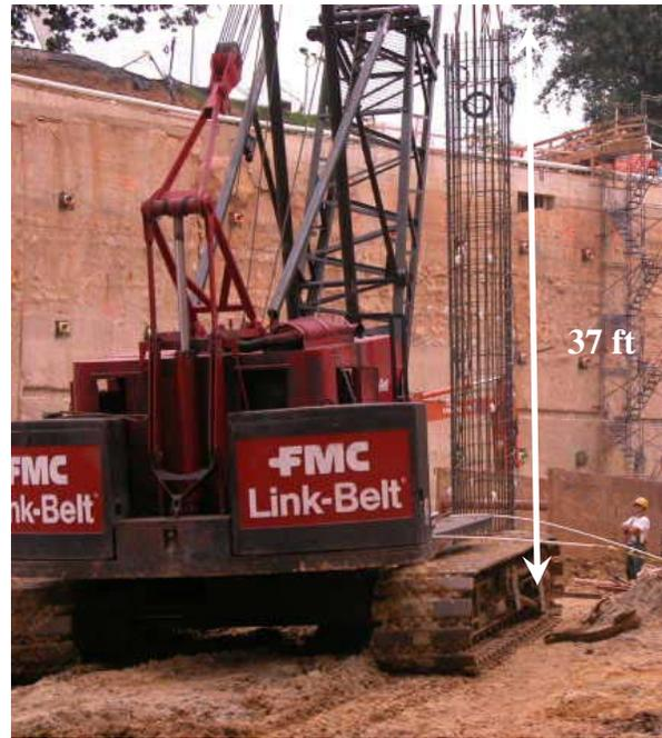
Figure 6 – Drilled Shaft Reinforcement
