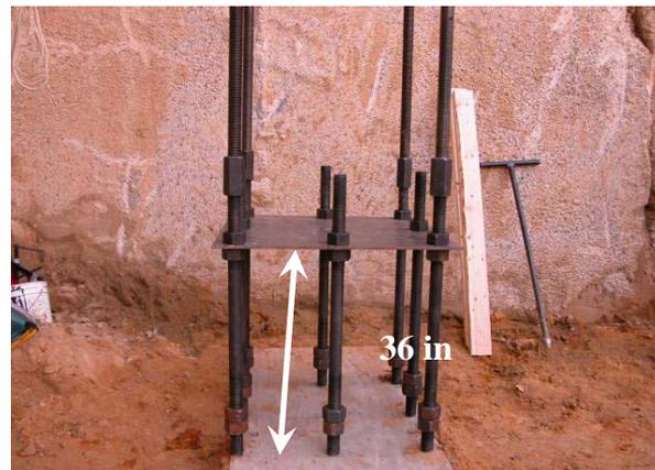
Figure 7 – Template of Embed Bars
