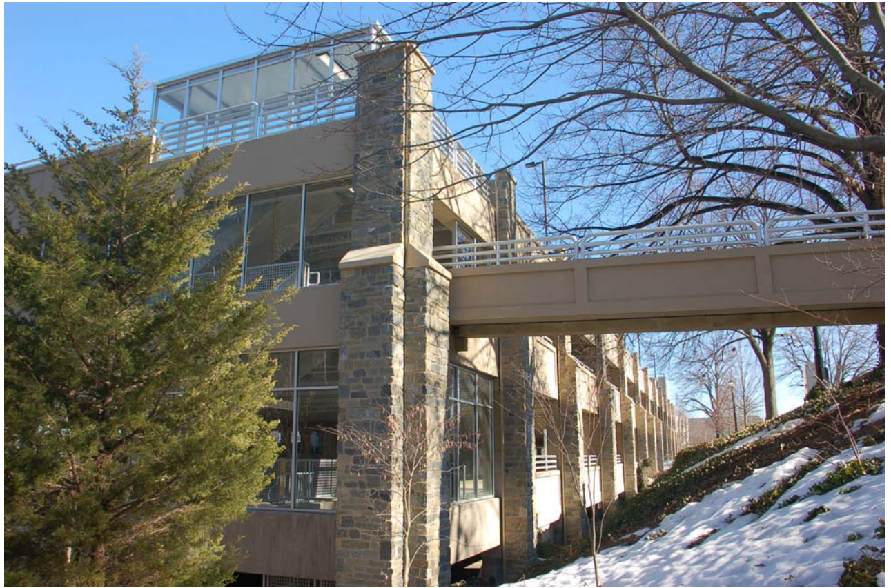
New Pedestrian Bridge
