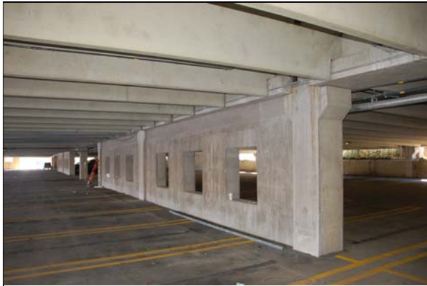
New Cast in Place Concrete Shearwall
