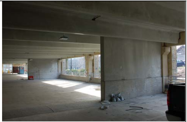
New Cast in Place and Precast Shearwalls at Perimeter
