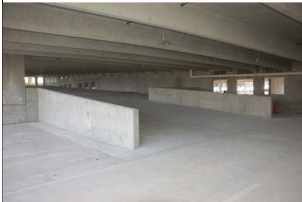
New Ramp to Access New Upper Levels
