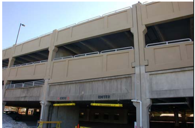
New Ramp to Existing Garage Interface
