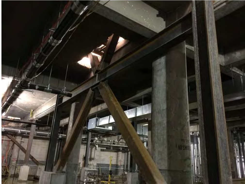
NEW BRACED FRAME BELOW EXISTING GROUND LEVEL
