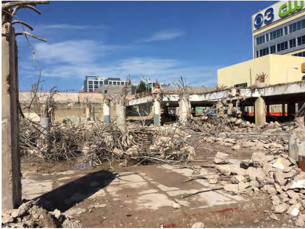
EXISTING STRUCTURE DEMOLITION ABOVE GROUND LEVEL
