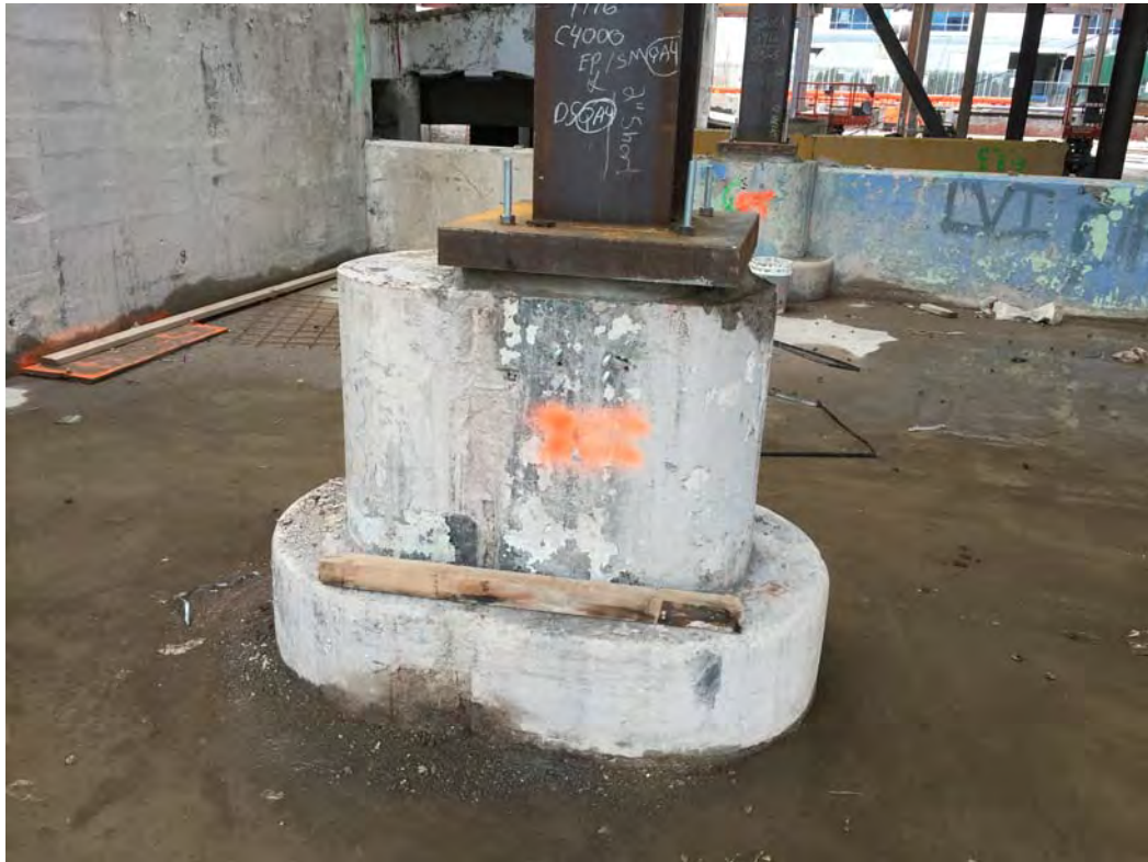
NEW COLUMN SUPPORTED ON EXISTING COLUMN STUB ABOVE GROUND LEVEL
