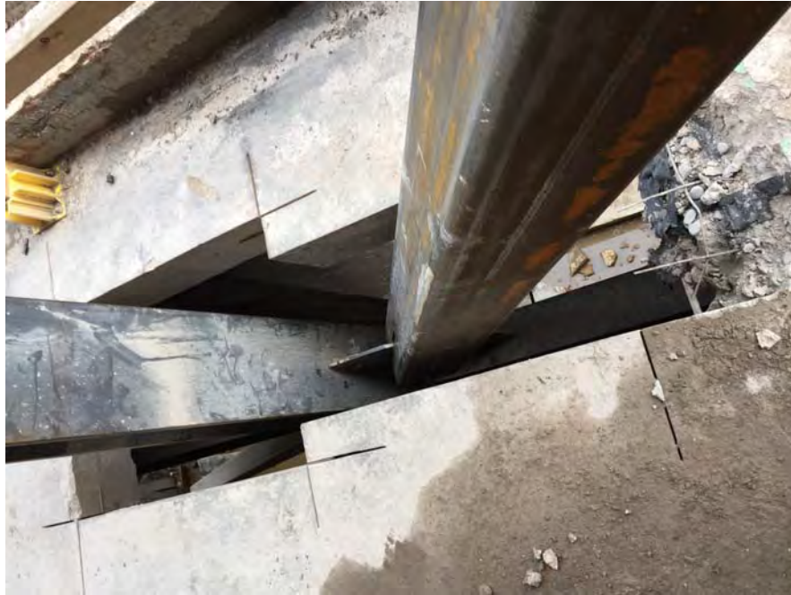
NEW BRACE / COLUMN THROUGH GROUND LEVEL SLAB
