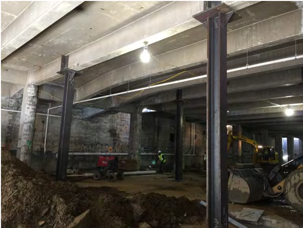
NEW STOP / START COLUMNS BELOW GROUND LEVEL
