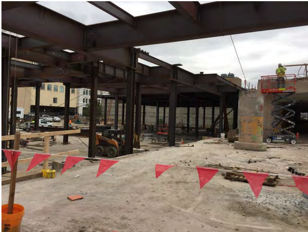
PODIUM TRANSFER LEVEL LOOKING SOUTHEAST
