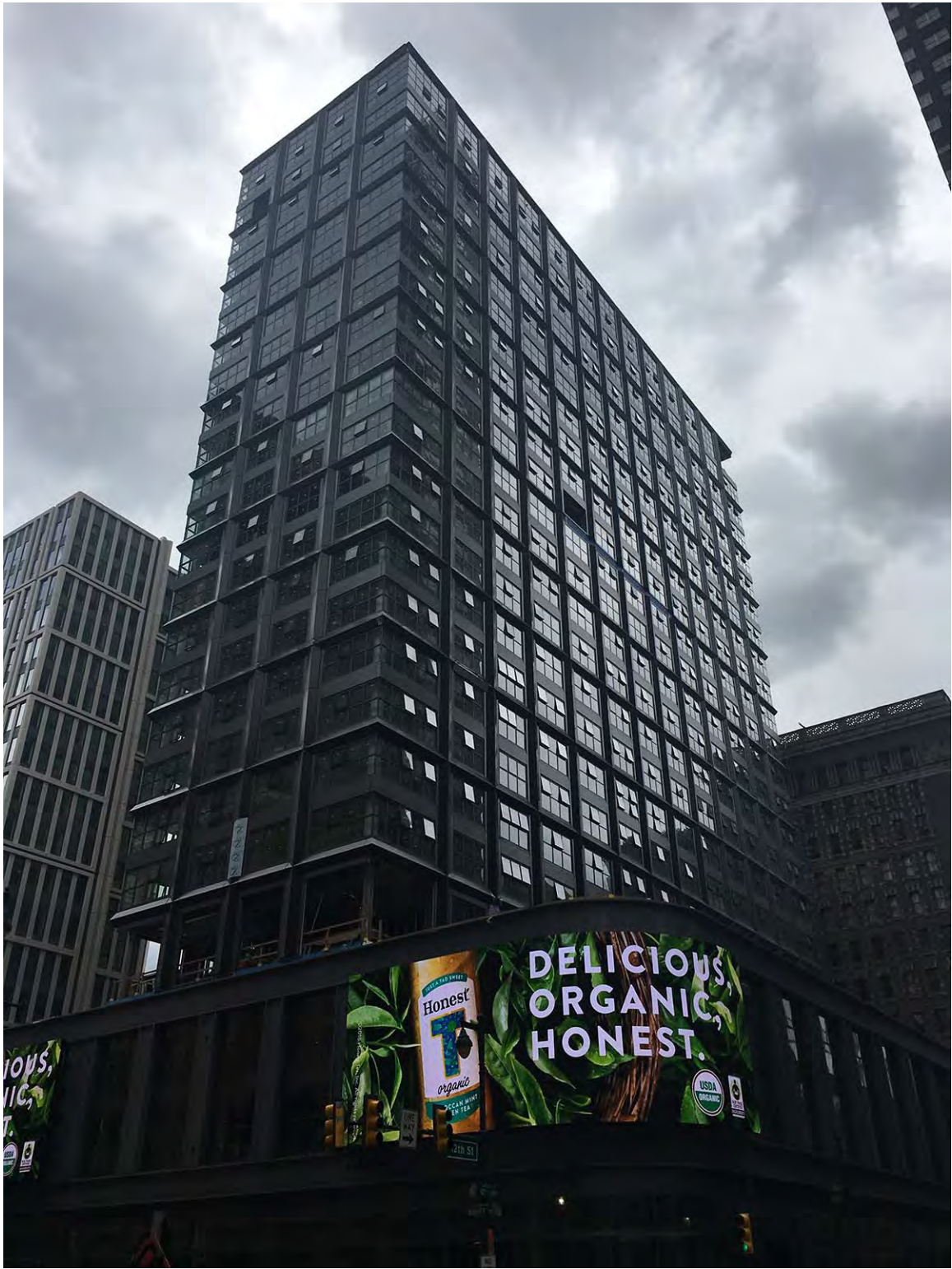
Phase 2 tower nearing completion
