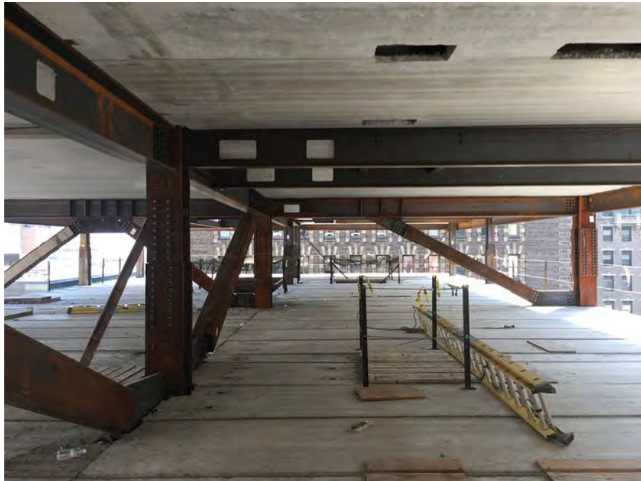
Phase 2 – Note eccentric braced frame to accommodate the central corridor as well as the beam penetrations to allow utilities to run in the corridors.
