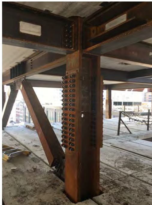
Phase 2 braced frame column splice at the 4 th floor. Note beam penetrations for getting utilities into the units.
