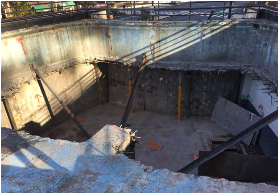
Demolition of existing pool structure. Exterior pool walls remain.
