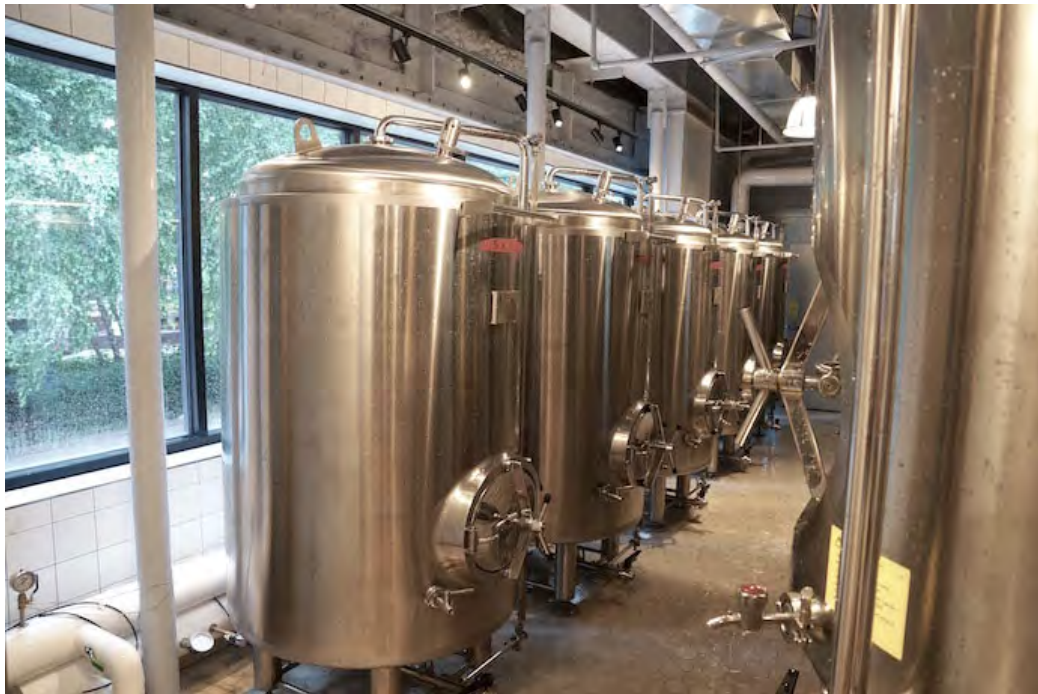
Addition of steel hangers to accommodate increased load from the production brewing system.
