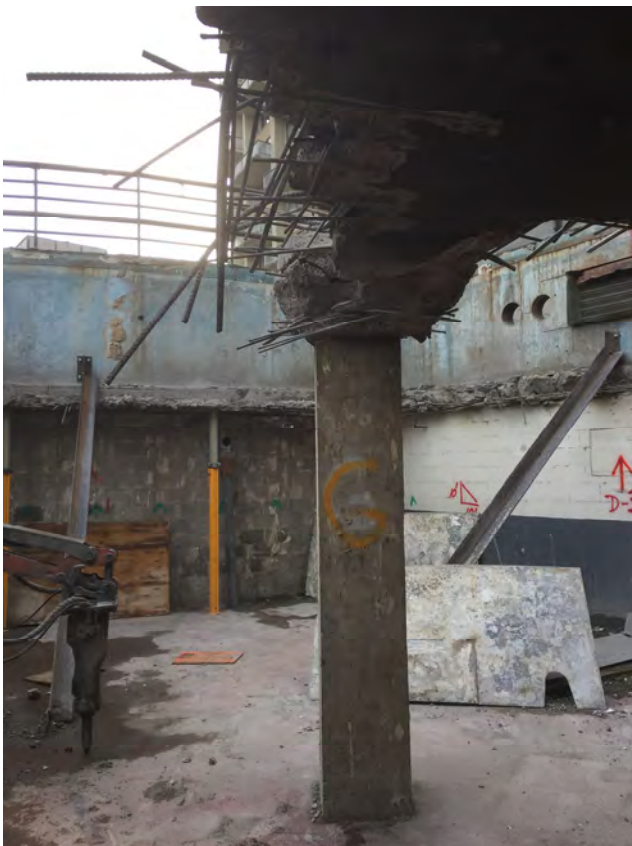
Demolition of existing pool structure. Exterior pool walls remain.
